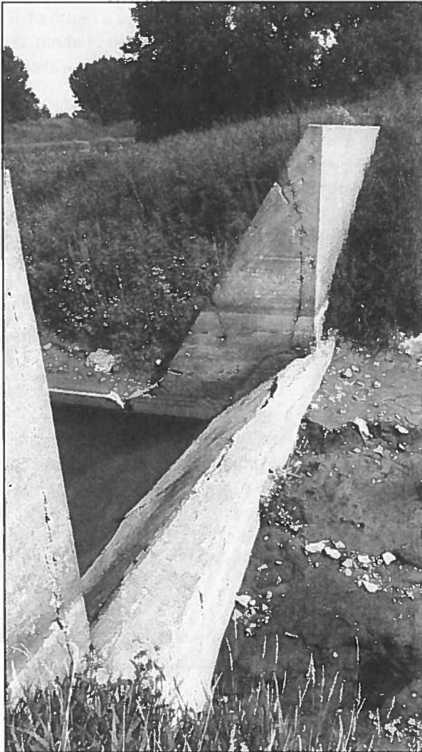
Photograph 2. Looking north at existing structure
