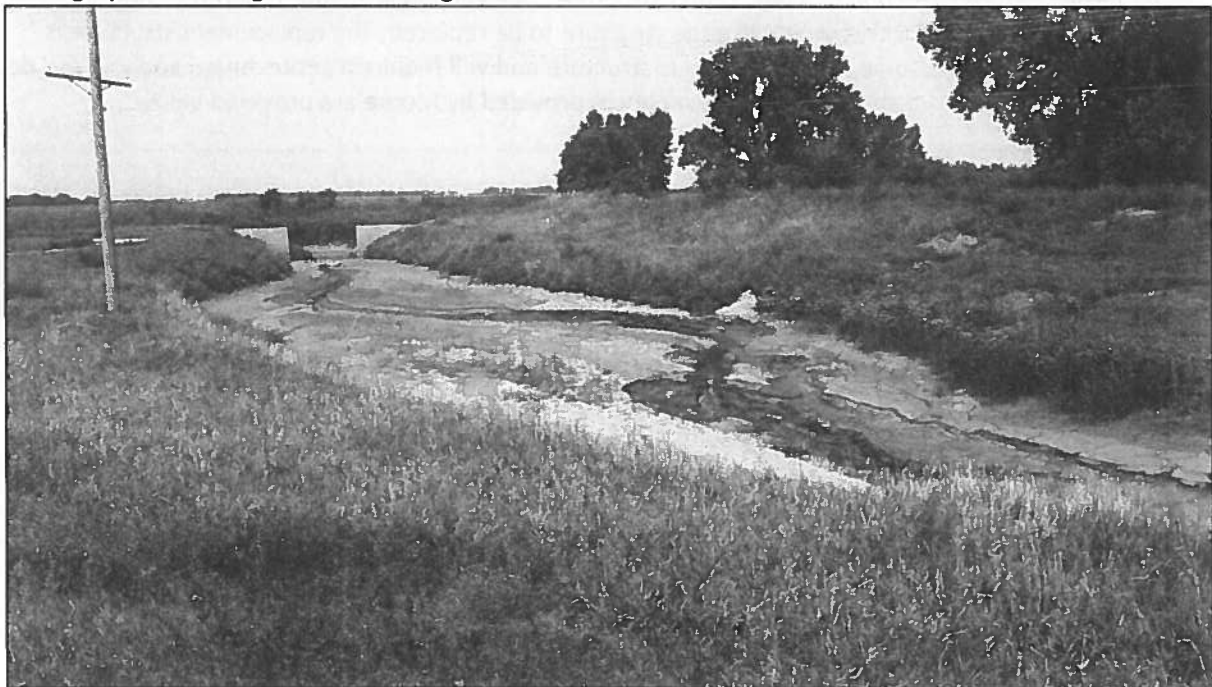
Photograph 1. Looking west at existing structure
